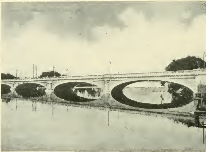
JEFFERSON STREET BRIDGE, SOUTH BEND.
